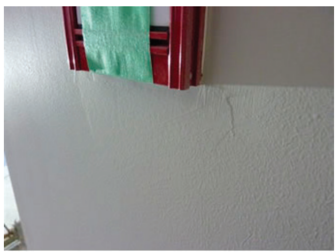
Brush marks from touch-up plainly visible on a rolled wall
